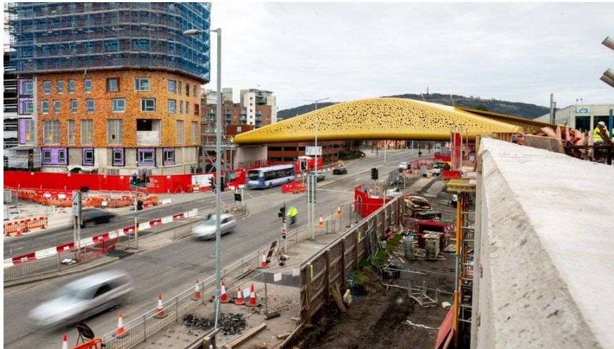
Figure 16 BBC (2021) Swansea landmark bridge lifted into place
