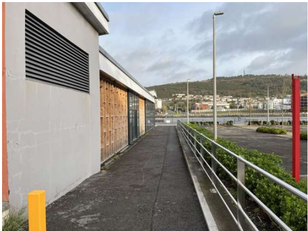
Figure 9 – Side of building off Kings Road
