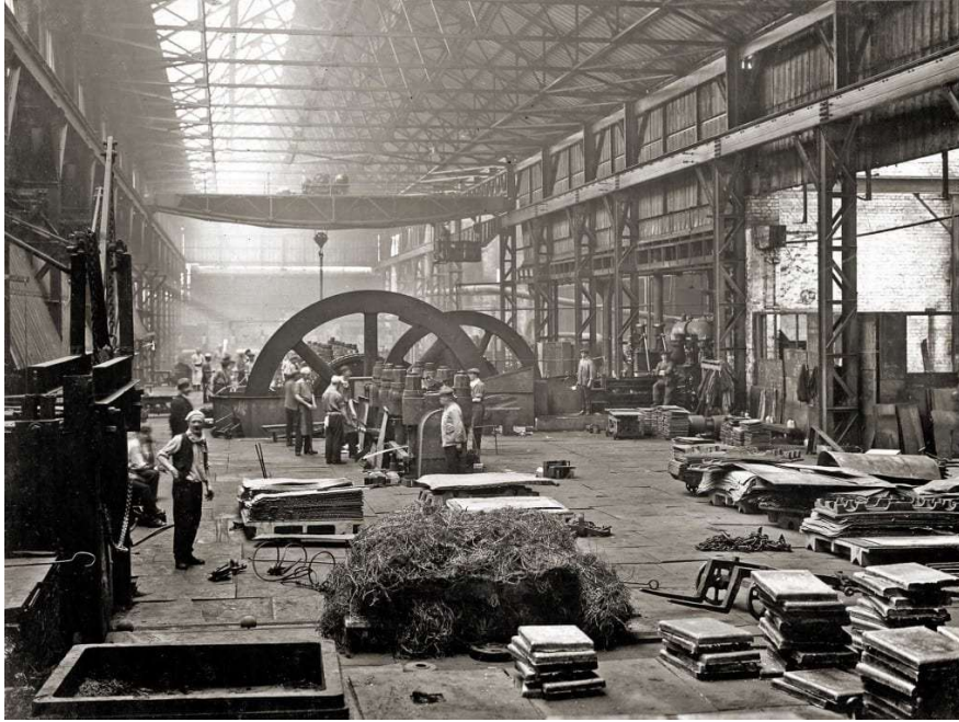
Figure 14 Gregory. R (2021) Work Progresses on Hafod –Morfa Copperworks Site
