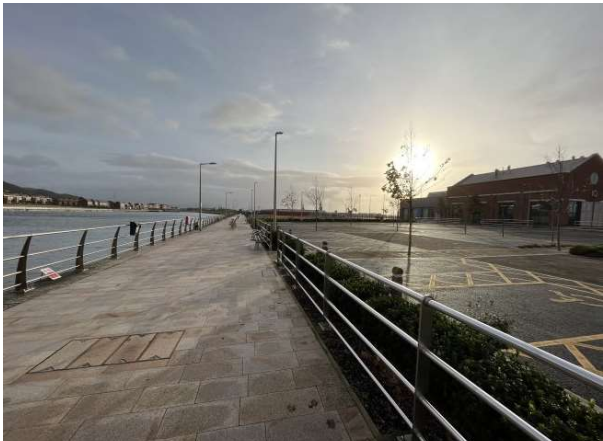
Figure 12 – Footway along Prince of Wales Dock
