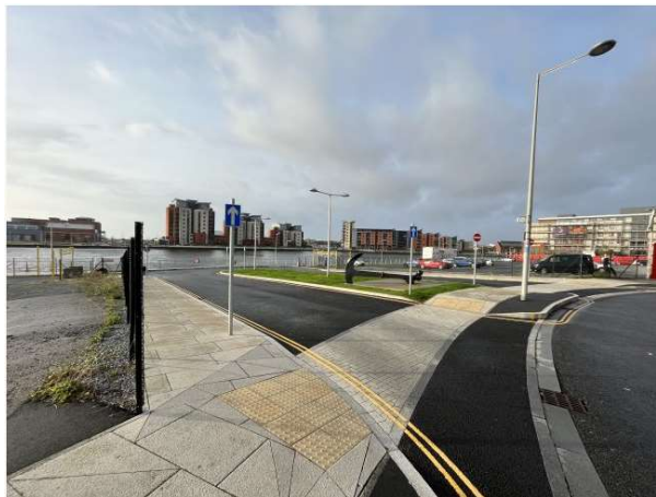
Figure 3 – Vehicle Access off Langdon Roundabout
