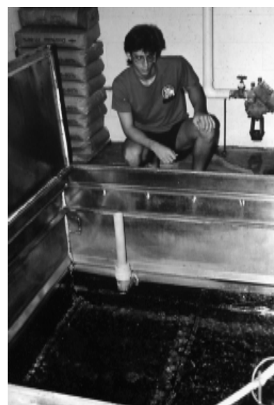
Fig. 5-5. Wet and dry wells for vacuum sand filters. (Photo courtesy of Tim Gervinski.)
