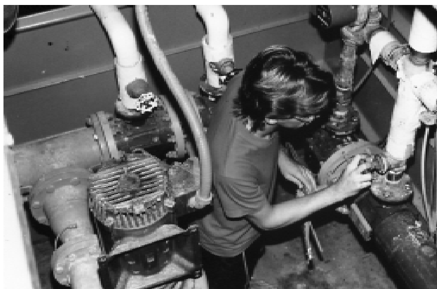
Fig. 5-5. Wet and dry wells for vacuum sand filters. (Photo courtesy of Tim Gervinski.)
