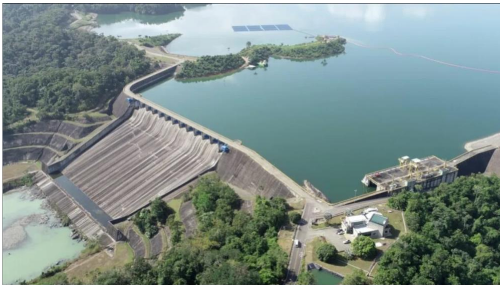
Figure 3. River Sinú Hydro-electric power station.
