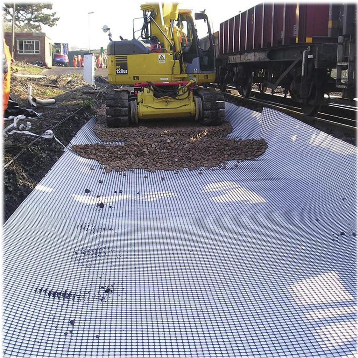
Figure 5: The implantation of Geotech© gridding suitable to reinforce weak sub-grade soils ( www.archiexpo.com , 2019).
