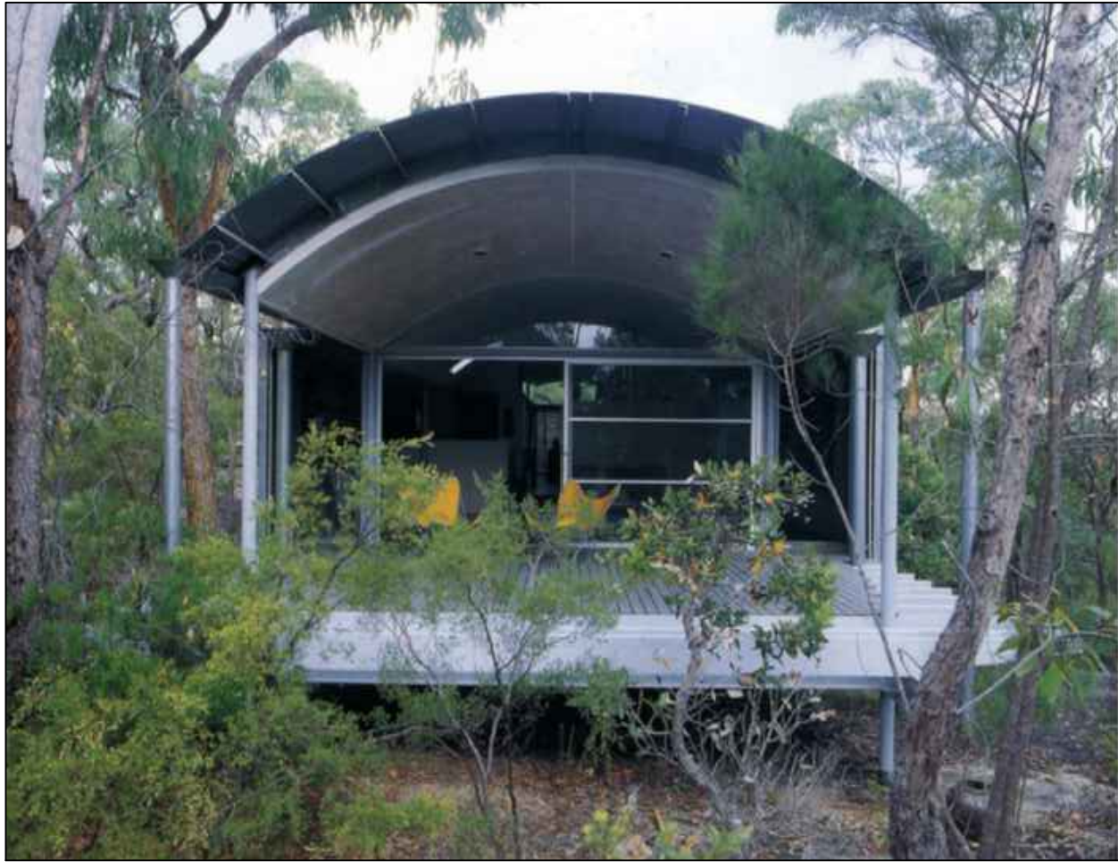
Image taken by Weebly (2018) https://balleastawayhouse.weebly.com/the-building
