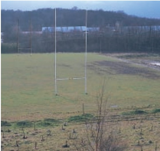
Lack of proper maintenance will exacerbate minor problems and eventually affect surface performance.
