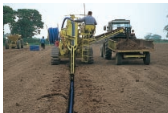
Installing pipe-drainage in a new pitch.
