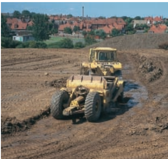
Many sites require major regrading of levels. Existing topsoil is removed and set aside for later use; level adjustments are made in the subsoil.
