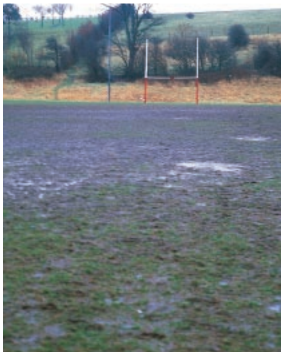
A poor quality pitch – appropriate planning, design, management and long-term maintenance are as critical to the success of a natural turf playing surface as they are to any other sports facility.
