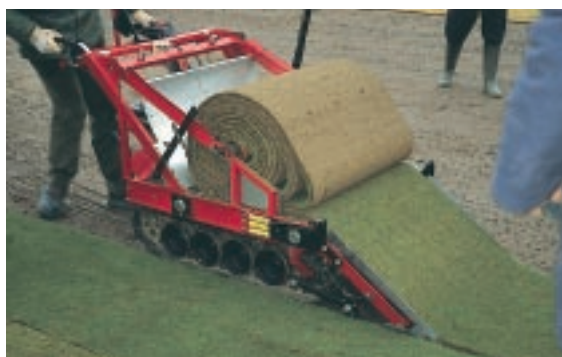
Laying wide roll turf.
