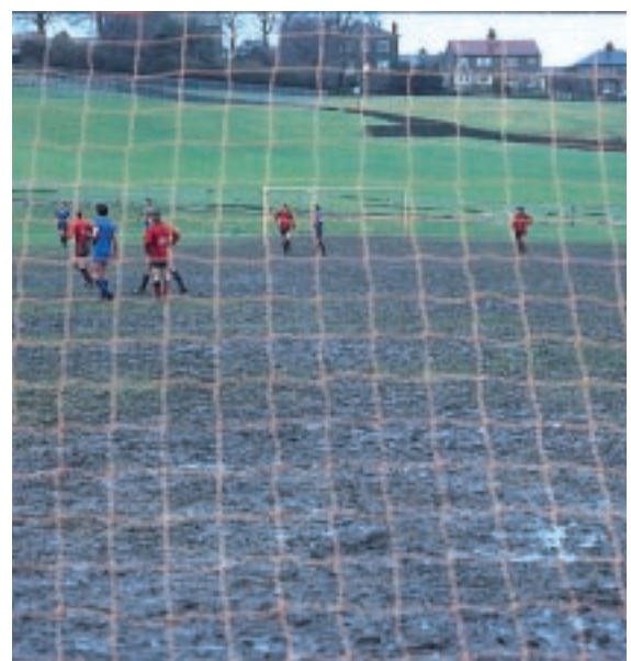
Badly constructed and maintained surfaces are dangerous and detract from quality of play.
