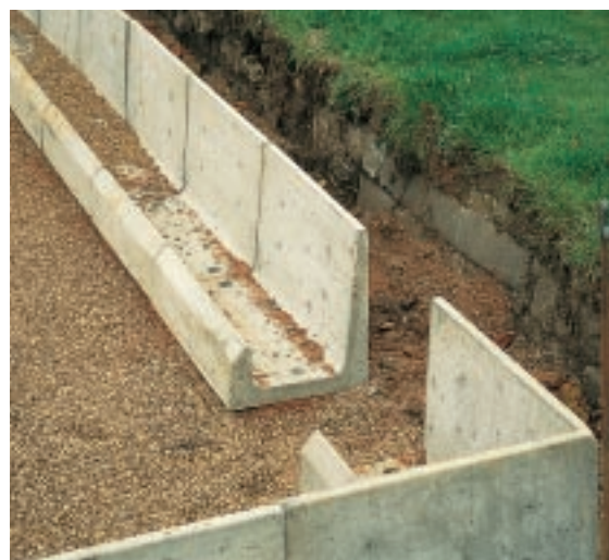
Pre-formed ditch channel simplifies construction.
