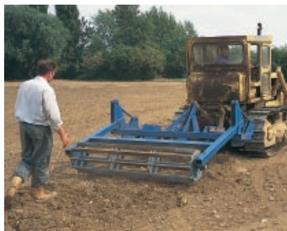
Cultivation of the subsoil is particularly important after major regrading.
