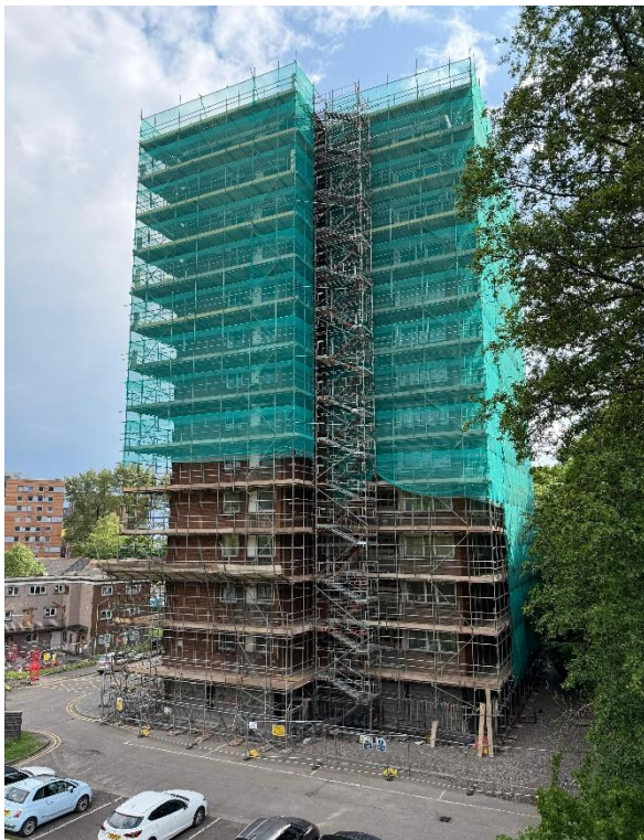
Figure 1. Residential Building, Croft Street Block 2, Dyfatty, Swansea. Source: Author's own photograph.
