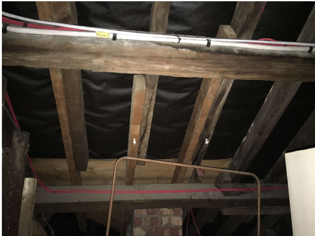
Figure 3.3.1: Internal image between rafters (Author, 2018)
