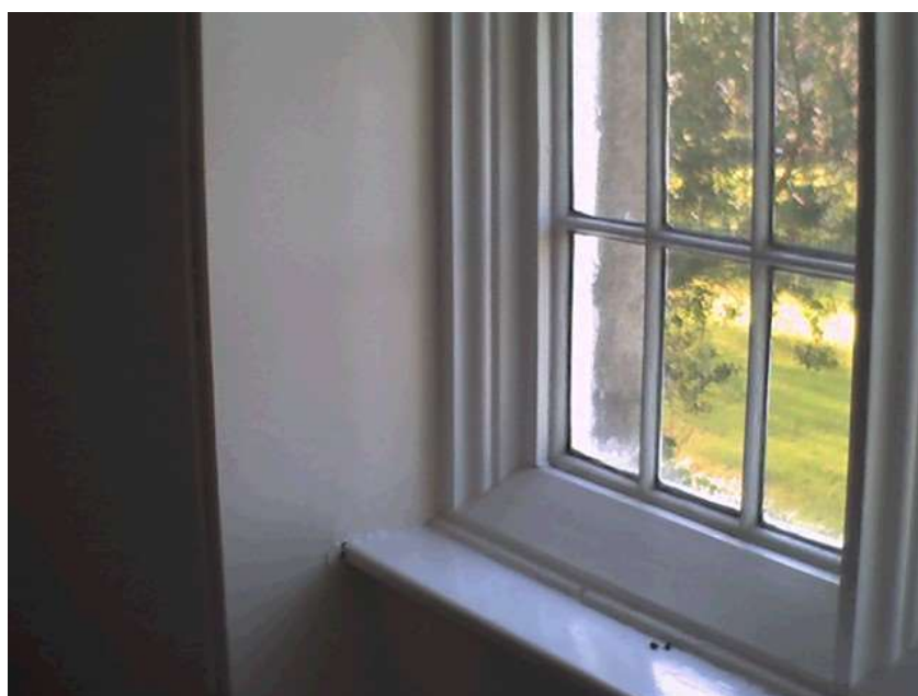
Figure 3.1.1: Internal image of existing timber window (Author, 2018)
