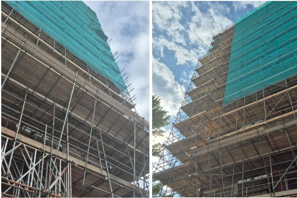
Figure 2. Site scaffolding and access controls at Croft Street Block 2 refurbishment project (Author's own photograph, 2026).
