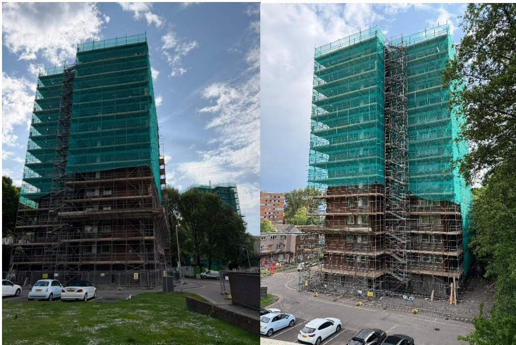
Figure 1. Croft Street Block 2 during refurbishment works in Swansea (Author's own photograph, 2026).
