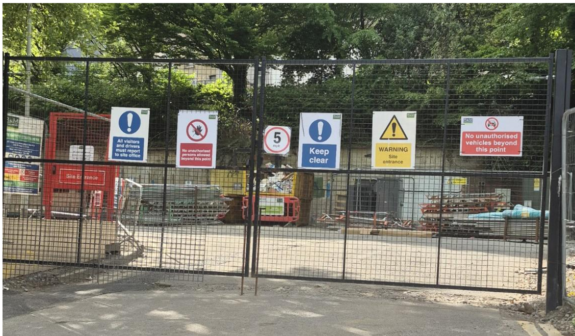
Figure 5. Construction site fencing and safety signage at Croft Street retrofit project (Author's own photograph, 2026).
