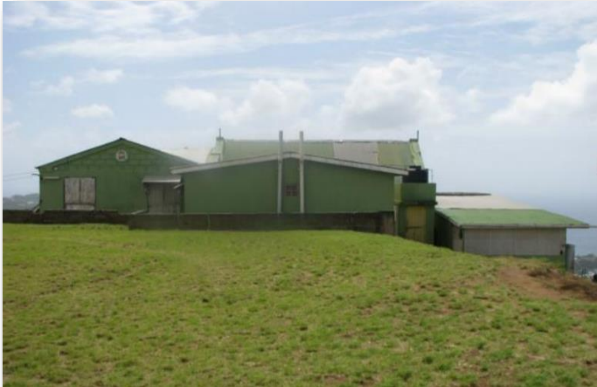
Picture 3: DHGS structure (rear view) before the SVG Regional Disaster Vulnerability Reduction Project that upgraded the school to an emergency shelter.
