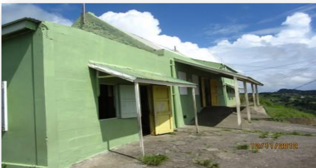
Picture 2: DHGS structure (front view) before the SVG Regional Disaster Vulnerability Reduction Project that upgraded the school to an emergency shelter.
