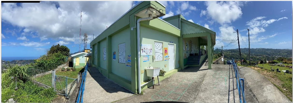
Picture 20: View of the DGHS mainbuilding and surroundings.
