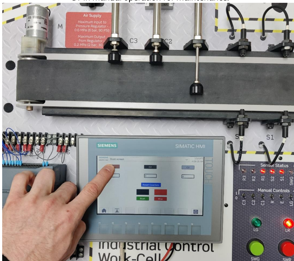
C1 in manual operation for maintenance.
