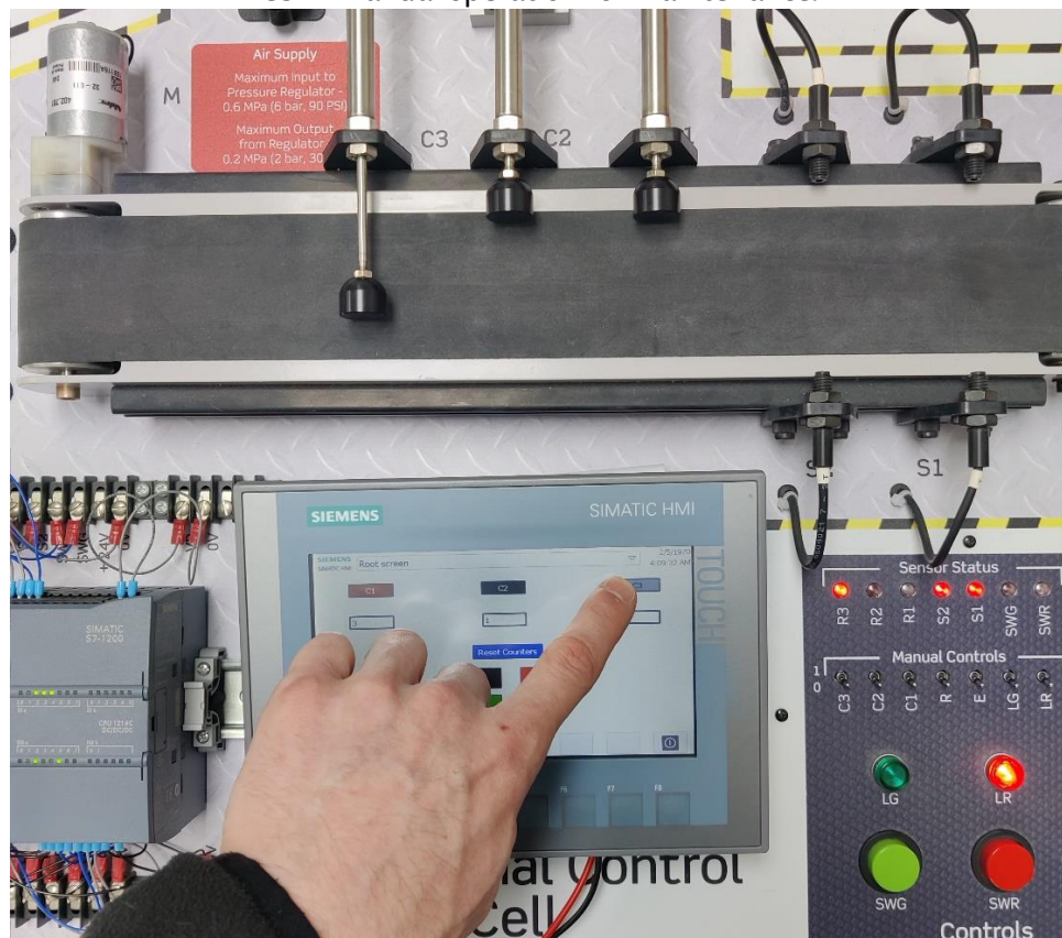
C3 in manual operation for maintenance.
