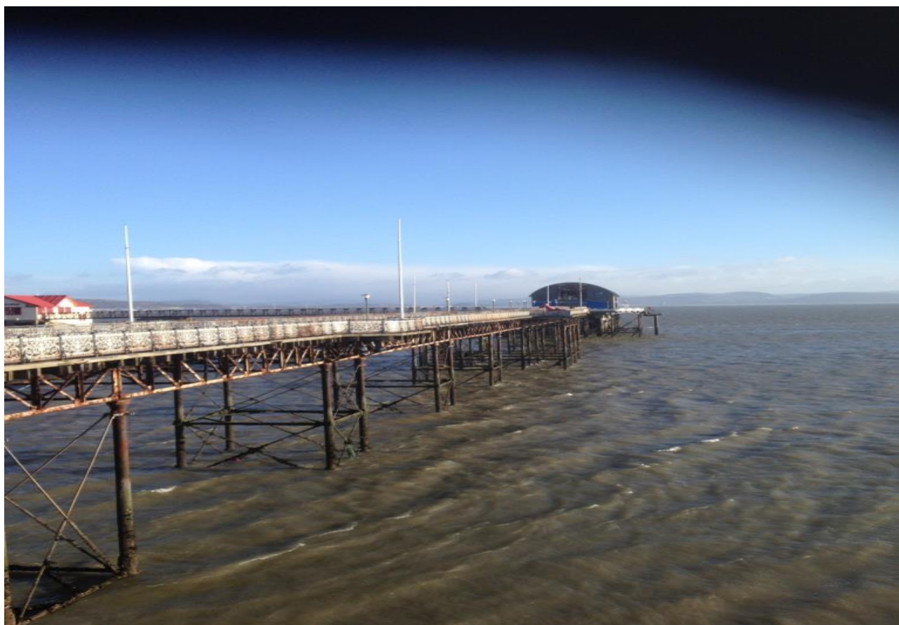
Image B: New Mumbles lifeboat station taken on 10 th January 2018.
