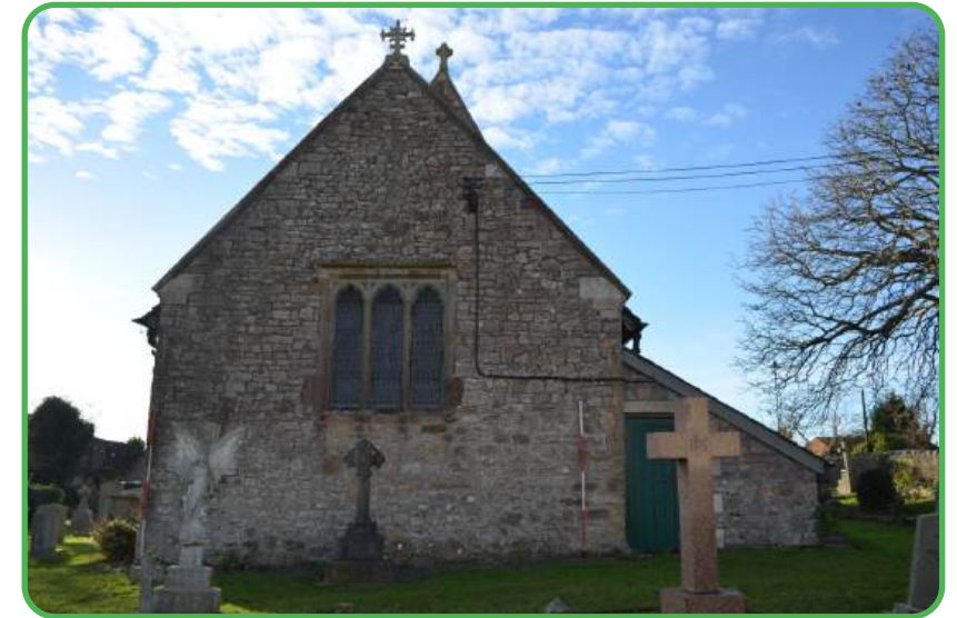
West elevation of St. Marys Church, Undy
