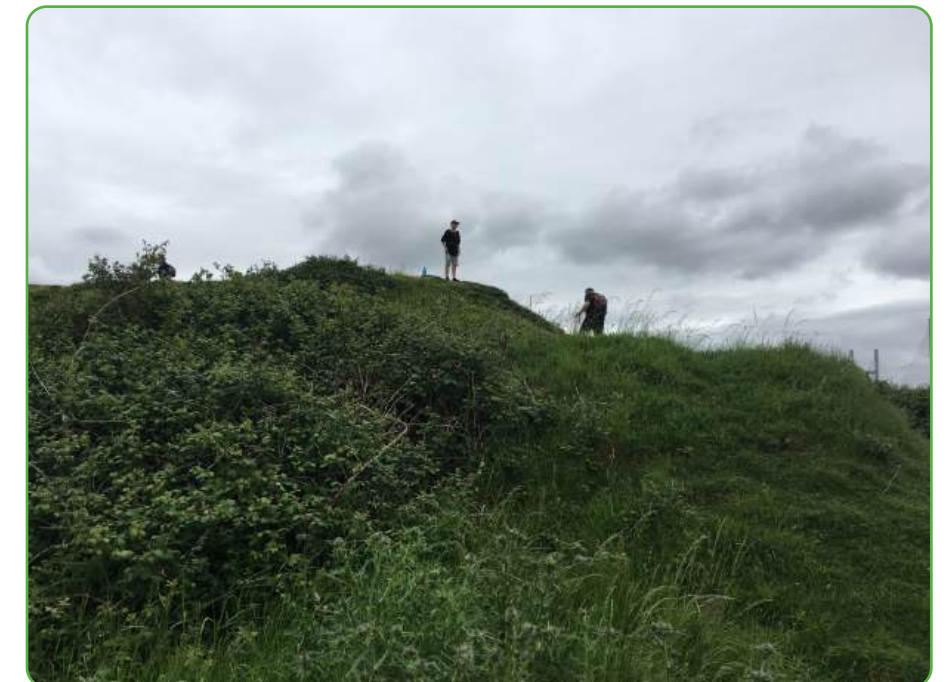
Lann, Tadhg investigate the Iron Age hillfort, Sudbrook Camp, and identify it as being under threat of continuous erosion from the sea
