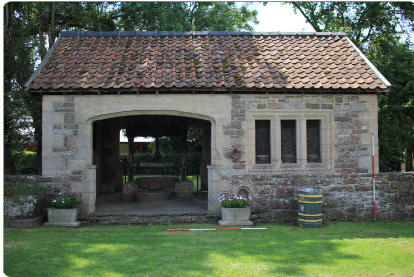
Front elevation, looking south, 2m scales
