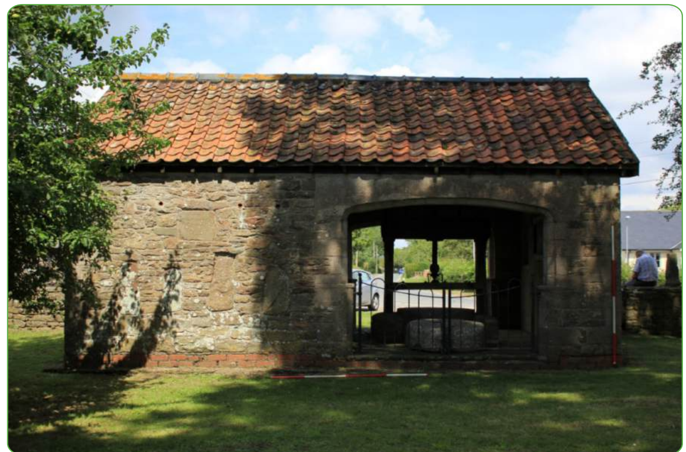
Rear elevation, looking north, 2m scales
