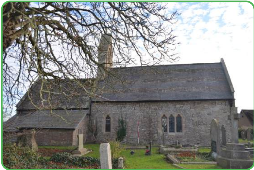
South elevation of St. Marys Church, Undy
