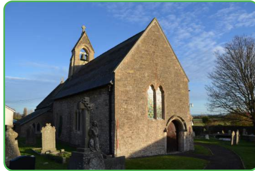
East and south elevation of St. Marys Church, Undy
