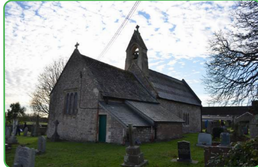
South and west elevation of St. Marys Church, Undy
