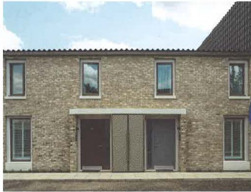
Goldsmith Street, the prize-winning council homes in Norwich
