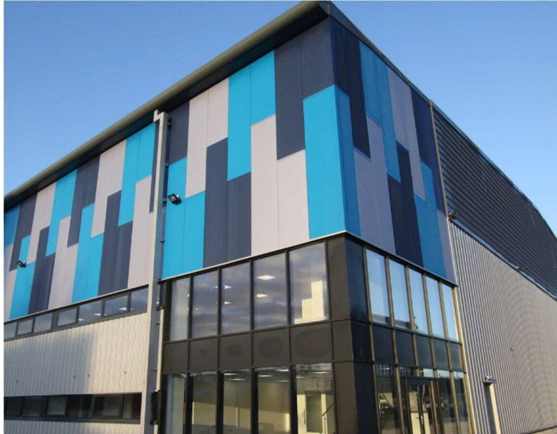
Figure 5 - Tata Steel UK. (2026). Trimapanel® insulated architectural wall panel systems.
