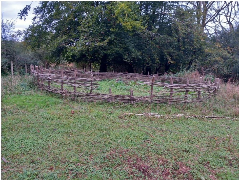
Figure 27: The finished fence of garden one from the new entry point (personal collection, 2024)
