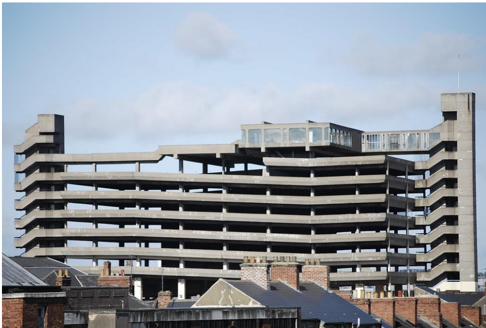
Figure 20: Trinity Square Car Park prior to its demolition. (Image: https://www.getcarter.xyz/ )
