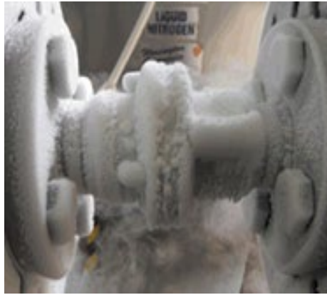
FIGURE 4: KLAW CRYOGENIC BREAK-AWAY COUPLING
