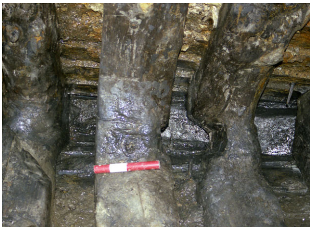
Figure 30. Roughly cut pump hole at F7/F8. (Nigel Nayling)
