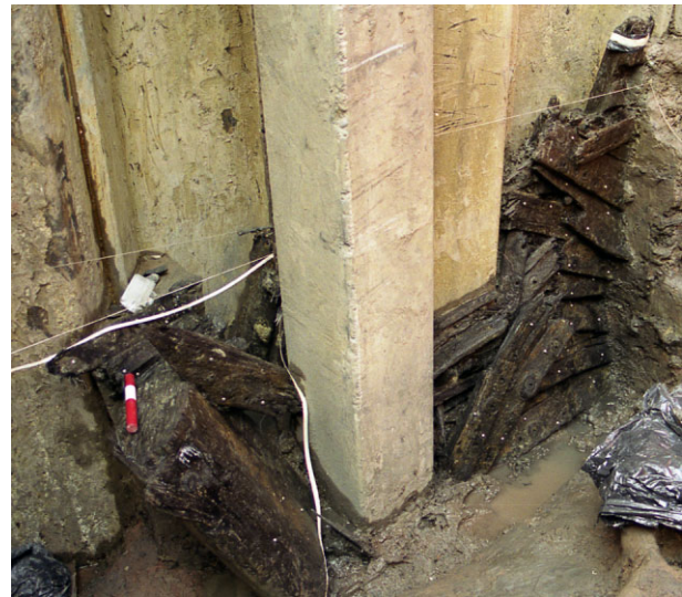
Figure 5. Excavation of the bow. View of outboard face of stem and associated forward hull badly disturbed by sheet and concrete piles. (Nigel Nayling)
