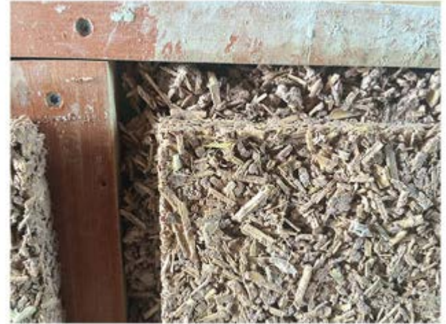
Panel interlock joint detail
