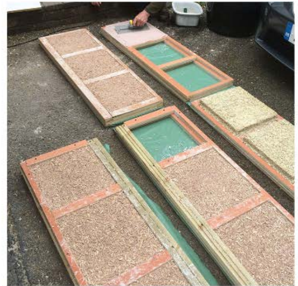
Finished panels laid out in mould ready for face coating of lime plaster
