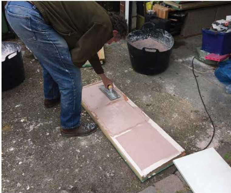
Finished panels of hydrated lime version finished with smooth lime plaster
