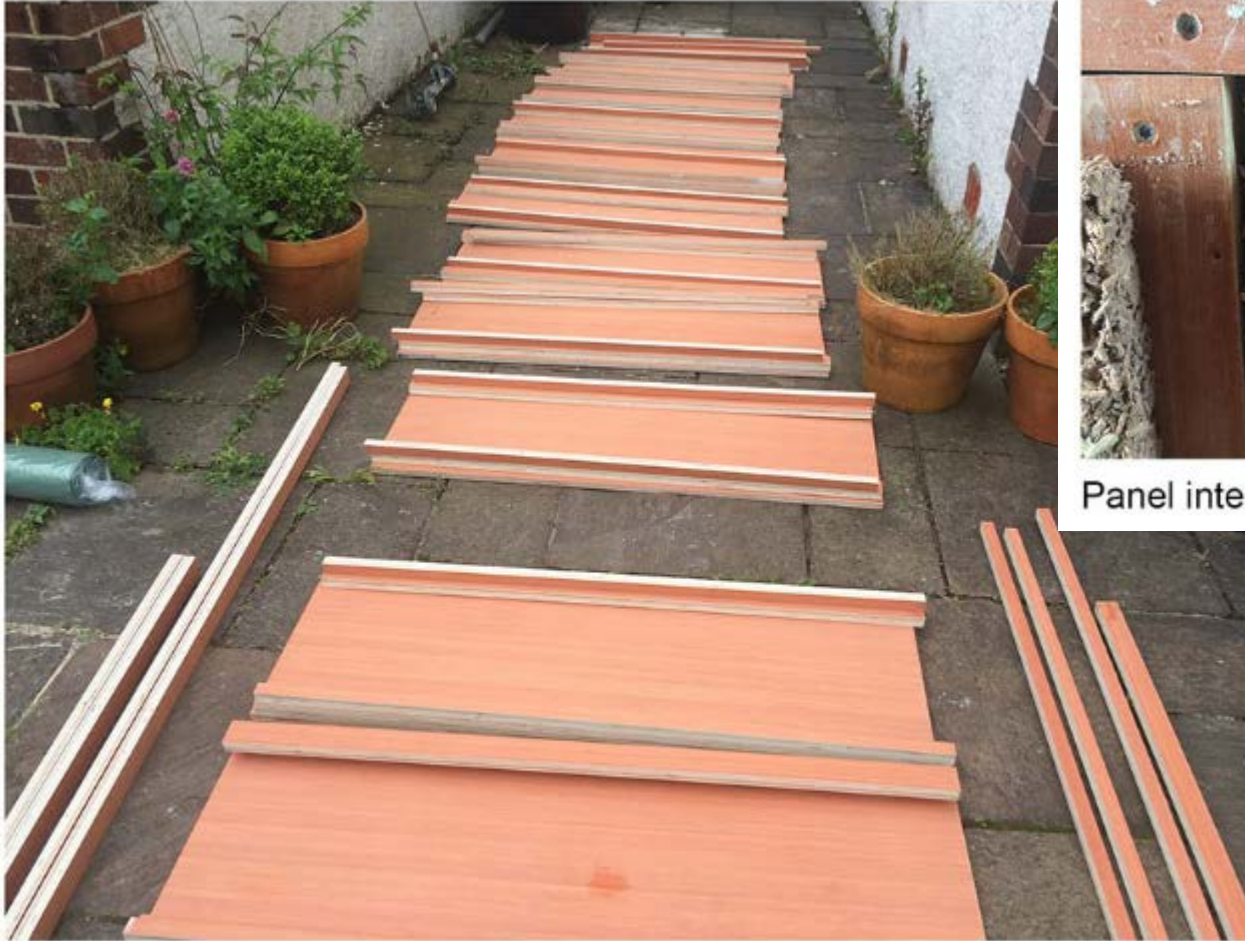
Modular plywood mould production with battens to form units
