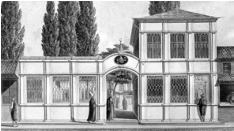
FIGURE 6.7 Front entrance to the Galata Mevlevi sufi lodge, early twentieth century.
