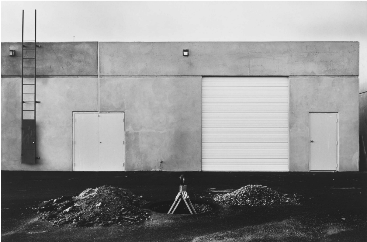
Fig. 2: Road Construction, Airport Loop Drive, Costa Mesa
