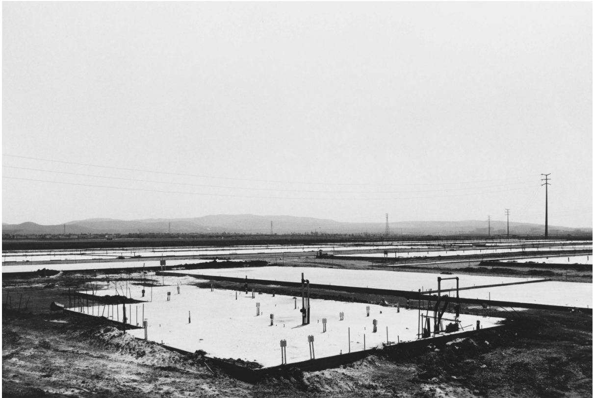
Fig. 1: Foundation Construction, Many Warehouses, 2892 Kelvin, Irvine
