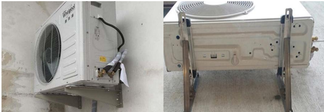
Figure 1. Supporting bar below in real case
