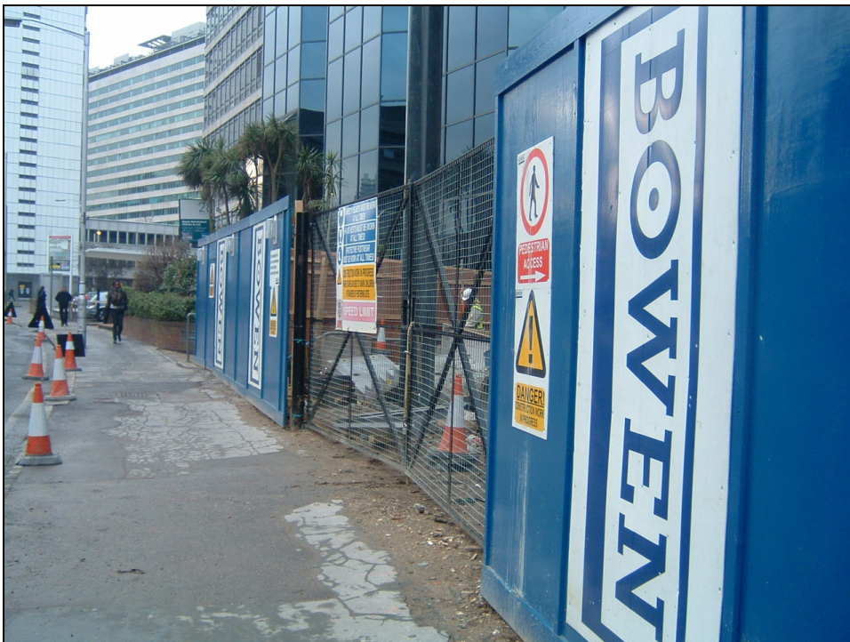
Photo shows 6m wide double access swing gate – gates swing into site.
