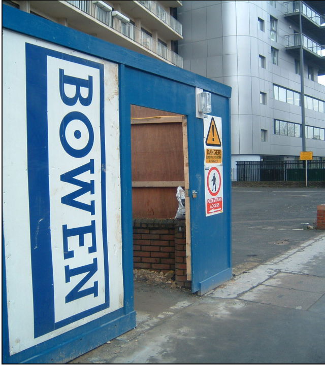
Photo shows single pedestrian access gate, which is locked during the night.
