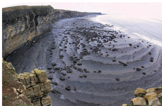
Figure 2 Section of the GHC looking east from Southerndown (site 34)
