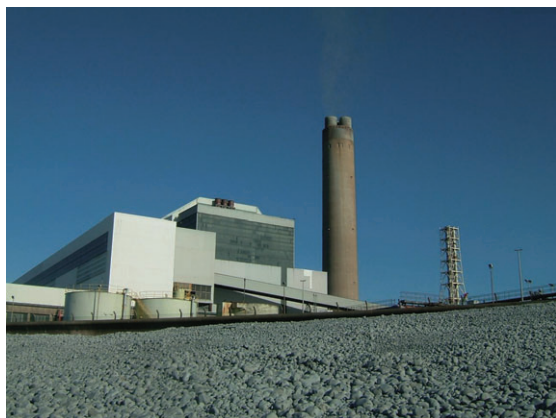
Figure 7 Aberthaw Power Station (site 1)
