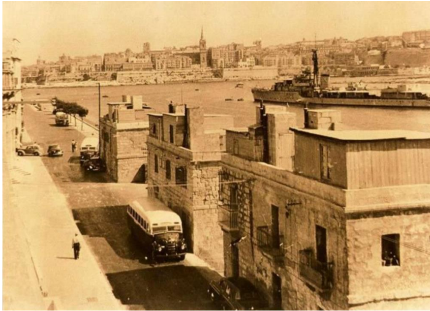
Fig. 5: Houses at the ferries in SLIEMA during the 1930s. Malta.
