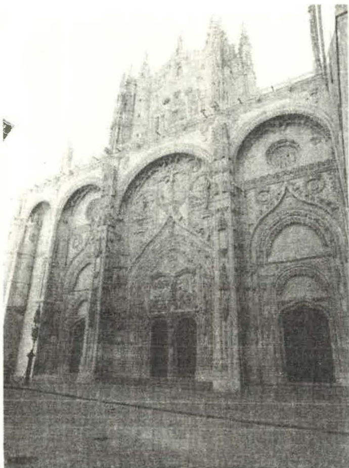
6. West Facade, New Cathedral of Salamanca, Spain.
