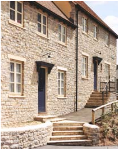
Coursed rubble stone - Thicket Mead, Robert Adam Architects
