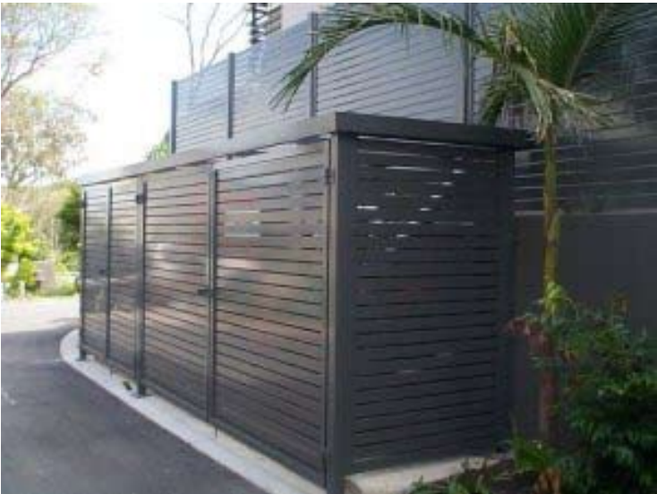
Booster pump enclosure
