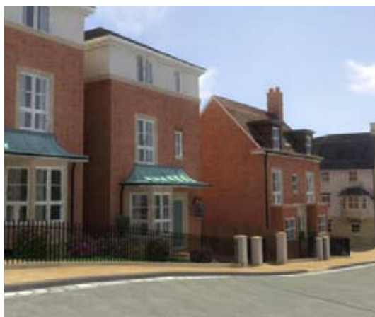
View along Middle Street
