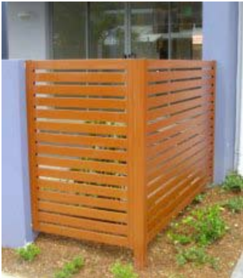
Timber look bin store
