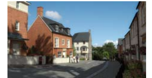
View along Middle Street
