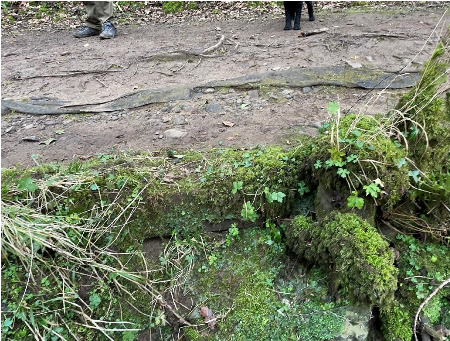
Figure 14 - Image showing soil erosion on footpath. (R Carter, 2022)
