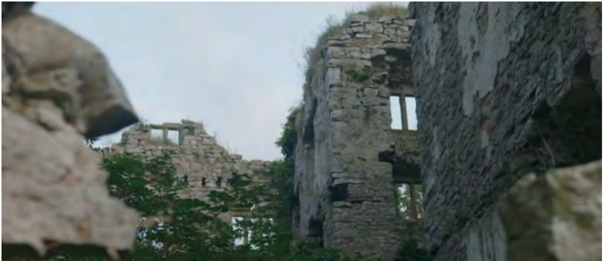
Figure 63 – View inside Foxhall, looking from ground level to roof level (Hidden Wales: Last Chance to Save, 2022)
