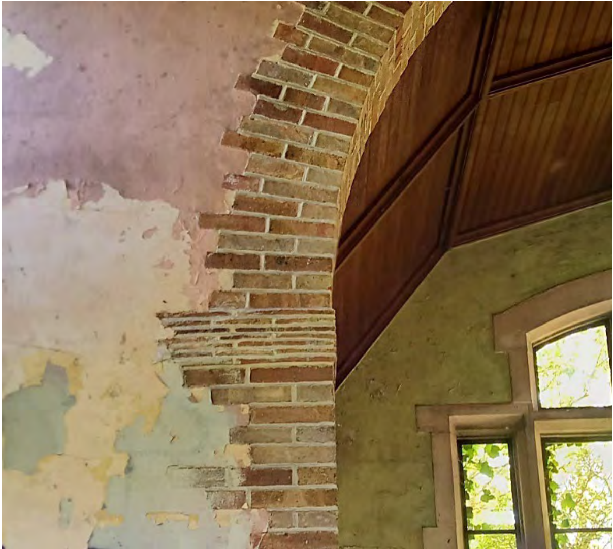
Figure 9 –Structural brickwork arch detail in the interior of the chapel (Author, 2021)
