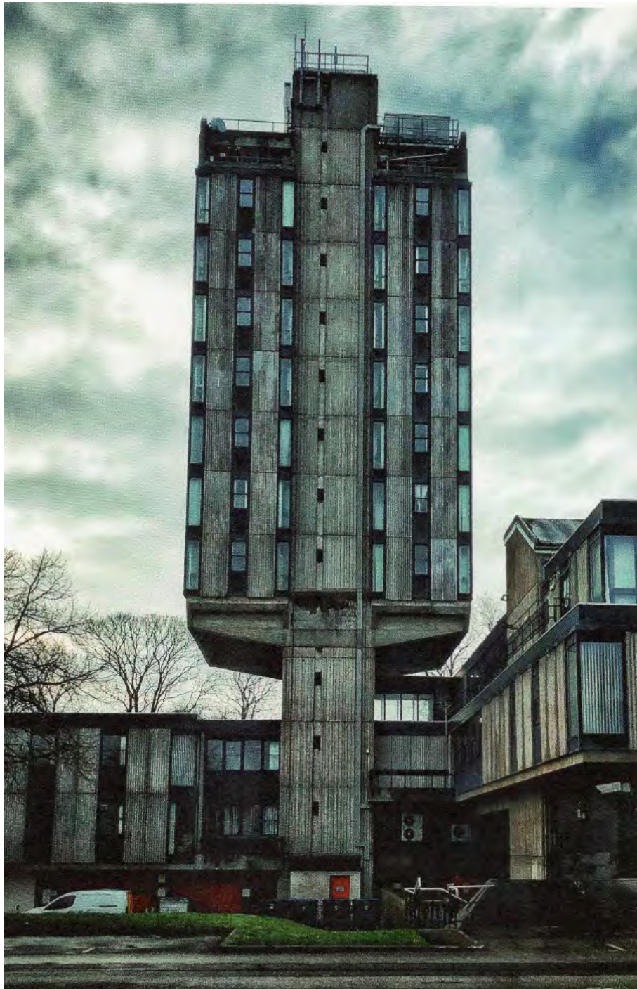
Figure 14 – Wrexham Police Station, 1975. (Halliday, 2021, p.15)
