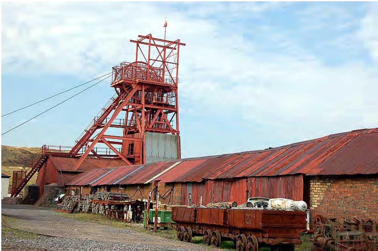
Figure 30 – Big Pit, Blaenavon – Tramway Sheds with repaired roof (Steinsky, 2006)
