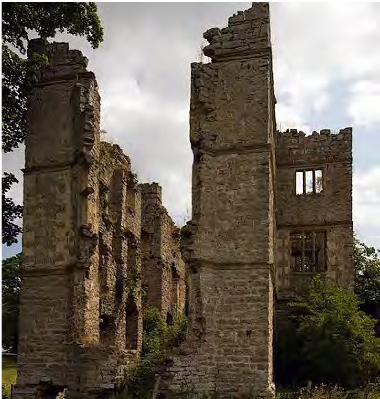
Figure 64 – View of Foxhall with missing façade large window (Seale, 2014)
