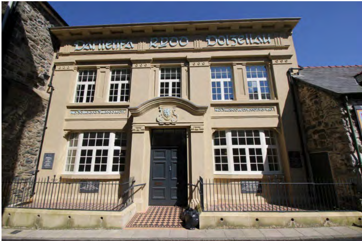
Figure 34 – Dolgellau Free Library building in North Wales, after renovation works (Buck, 2015)
