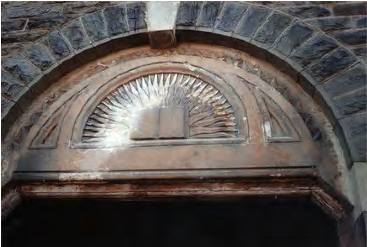
Figure 54 – Unique detail above gable end doorway depicting the sun behind the bible, now lost to time (D.Workman, 2008)
