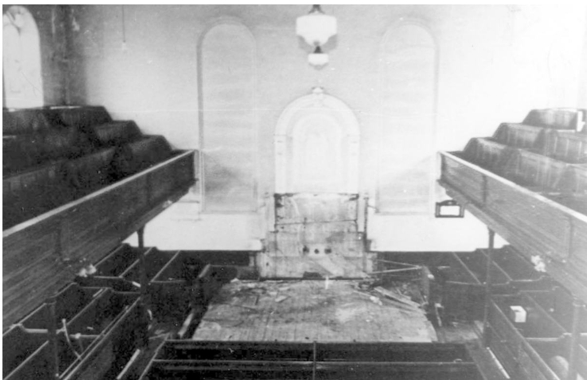
Figure 50 – Penuel Chapel interior view from balcony (RCT Digital Library Archive, 2020)
