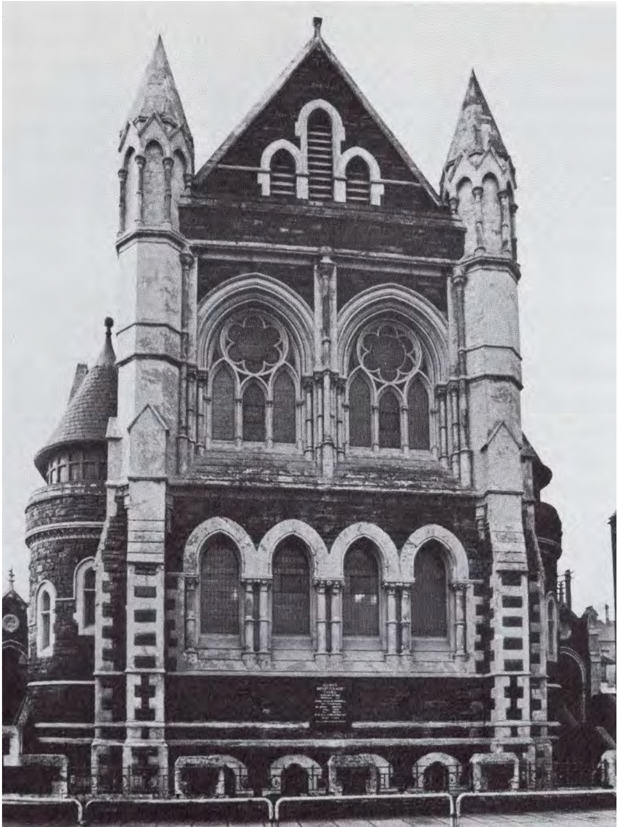
Figure 9 – Capel Pembroke Terrace, Churchill Way, Cardiff (H.C.Harris, 1877) (Hilling, 1973, p. 143)
