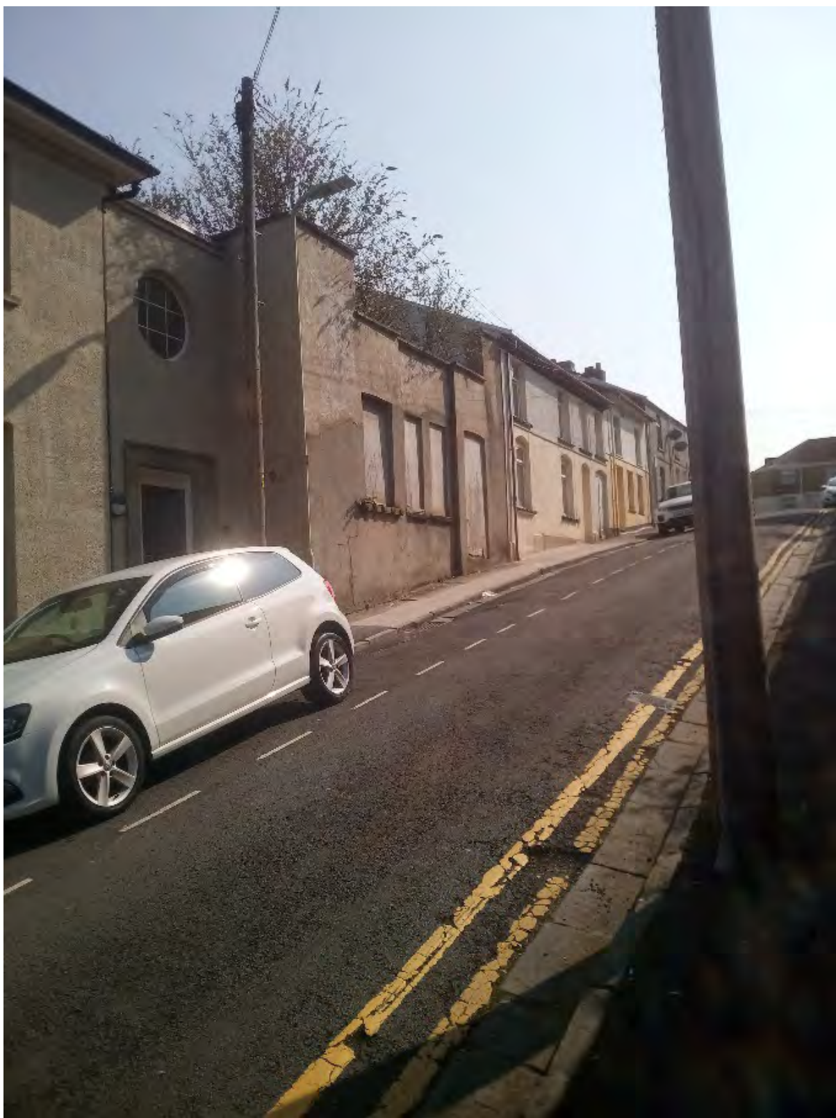
Figure 58 – Bethania Chapel Sunday School as existing, looking from north (Author, 2022)
