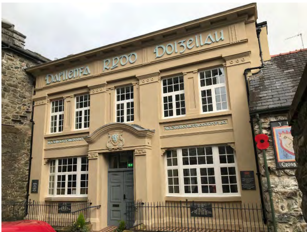
Figure 37 – Dolgellau Free Library with restoration of the original Welsh writing (Davies, 2015)
