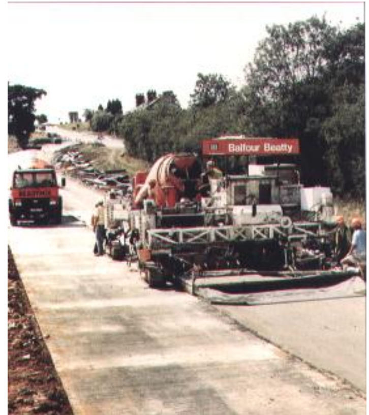
Compaction, curing and finishing
