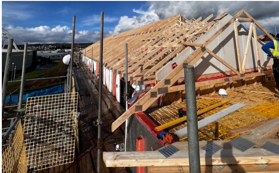
Progress Picture (Roof Truss cassettes Installation)
