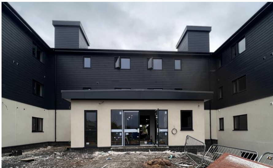
Progress Picture of front elevation (Main Entrance)
