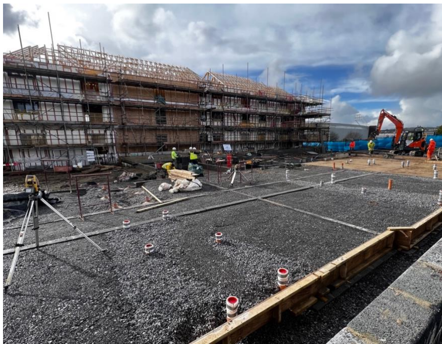
Progress Picture including partial timber frame erection and the construction of the Ground floor slab
