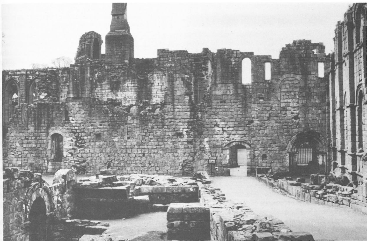
13 Part of Murdac's east cloister range survives to full height encased within a later rebuilding. It can be identified by its small, roughly-squared blocks of gritstone with wide mortar joints, the remains of thick external white-limed plaster, and with absolutely plain doors and windows detailed in good quality ashlar.
