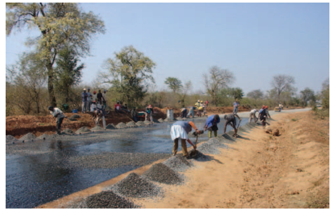
Labour-based sealing-spotting and spreading of aggregate
