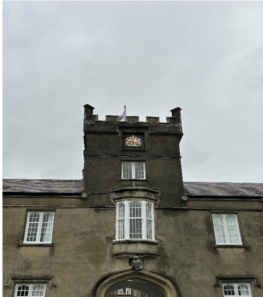
Figure 4 Showing the External Entrance Tower- Author
