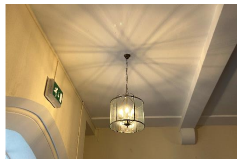
Figure 6 Showing Entrance Hall Lighting - Author
