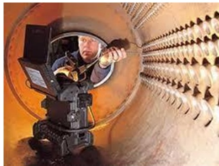
Figure 15. Visual NDT of a Heat Exchanger. (Olympus, 2019)
