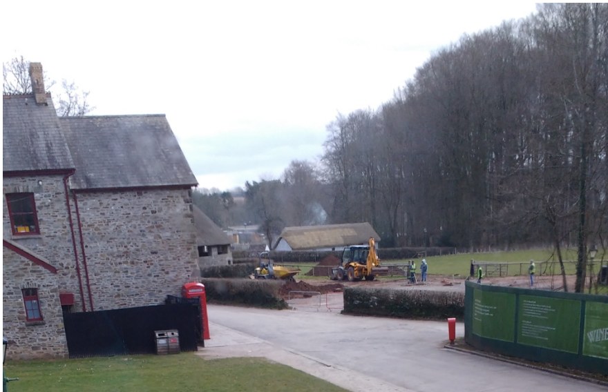
Image 5: Construction work of the Vulcan, image taken through the top window of the Workmen's Institute. My own image.
