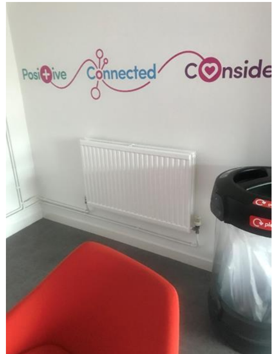
Plate 14: Typical heat source with localised control
