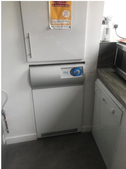
Plate 13: Typical gas fired heating system
