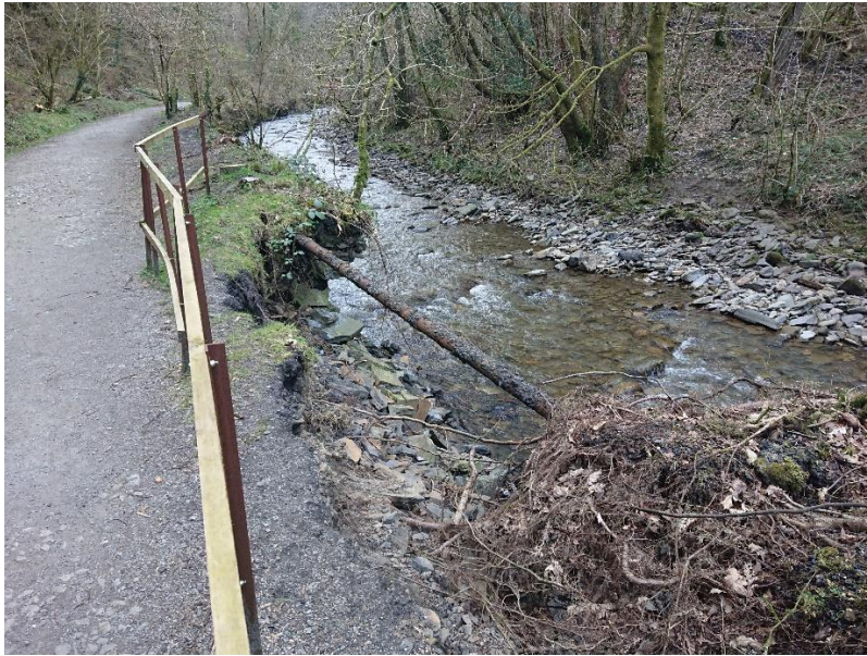
Figure 16: Further collapsing riverbank at location site, image author's own 2021
