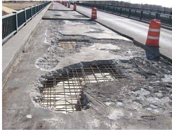
Figure 2: Concrete bridge deck patching
