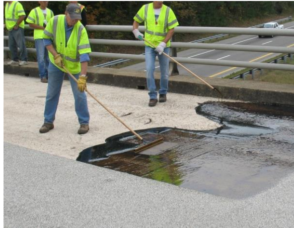
Figure 4: Concrete deck sealing
