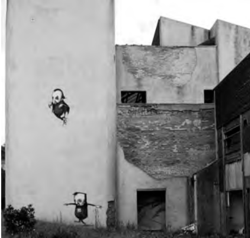
Figure 9.7 Two of Stormie Mills's characters moving towards the central courtyard at Pollphail. They are situated on the peeling render of a stair tower, adjacent to a piece by Derm, in a recessed doorway (Historic Environment Scotland DP246443).
