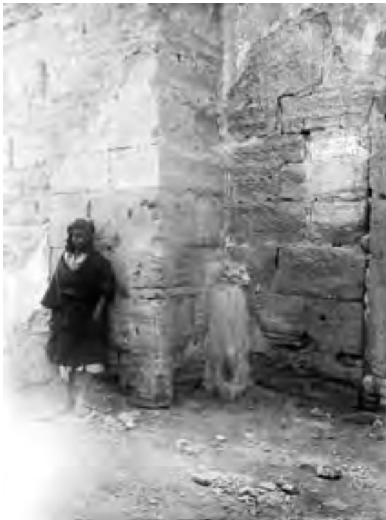
Figure 4.7 South interior wall of the Palmyrene Gate in 1928–1929. The doorway shown in Figures 4.1 and 4.6 is just out of the shot, its frame and inscription visible to the right. Just above the painted inscription the chalk label 'J16' is visible, part of the recording of the texts that lined the passageway of the gate. The name of the worker standing on the left is not recorded (Yale University Art Gallery, Dura-Europos Collection, scan of glass negative B27).
