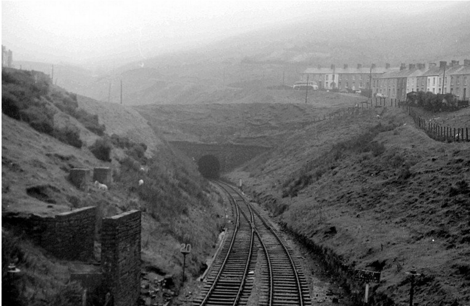
Figure 3: The Rhondda and Swansea Bay Railway Tunnel
