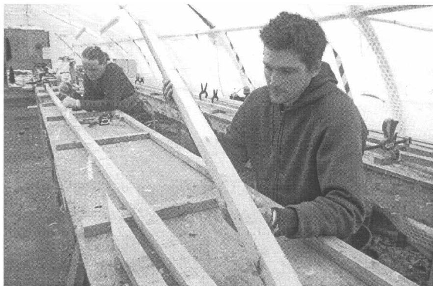
Figure 11 Construction of a scarf joint
