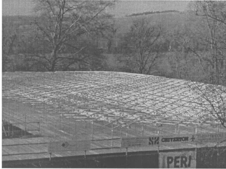
Figure 21 Completed layout of the flat lattice mat
