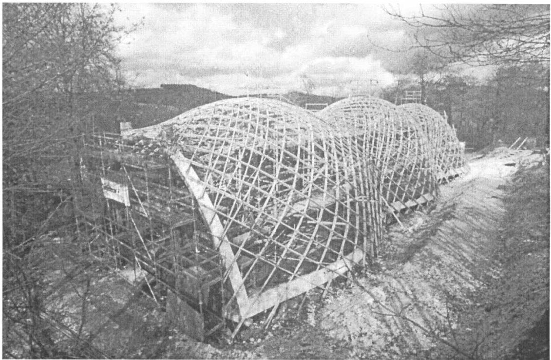
Figure 31 Final shape from the west platform
