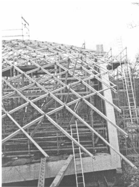
Figure 27 Gable end strapping system
