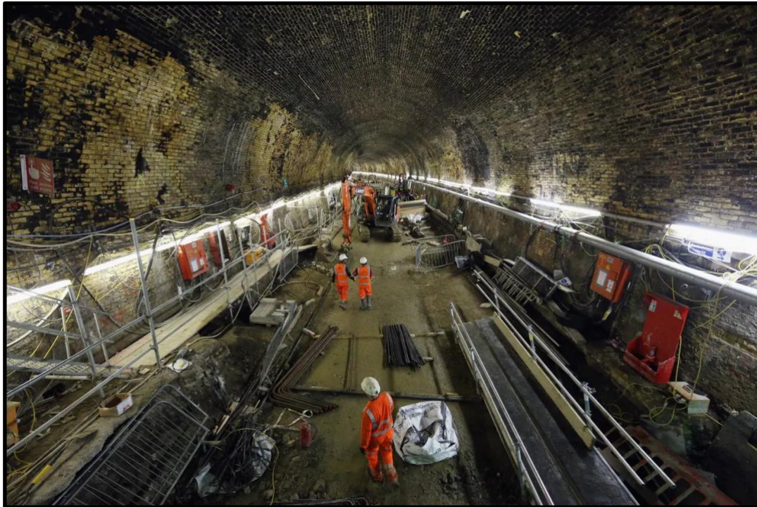
Figure 1: Tunnelling inside the Elizabeth Line
