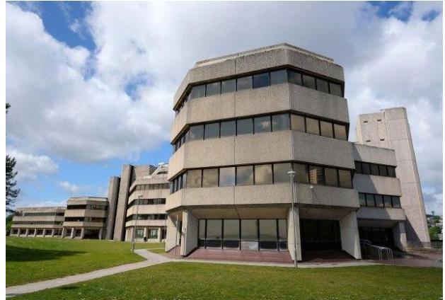
Figure 5 Coastal exposure of the Swansea Civic Centre, highlighting its vulnerability to adverse weather conditions. Source: Geograph Britain and Ireland.
