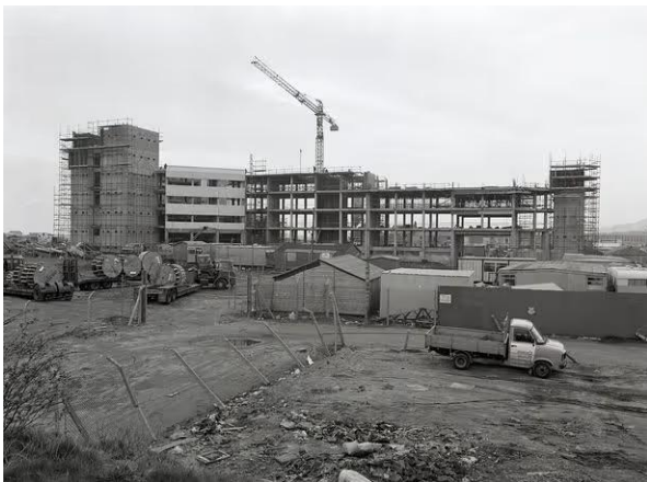
Figure 6. In situ concrete construction process showing formwork and labour-intensive methods, illustrating longer construction time compared to steel framing systems. Source: Walesonline.co.uk
