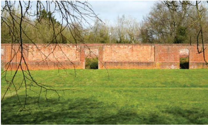
Figure 3.19 Showing embankment up to walled garden and reconstructed garden wall.
