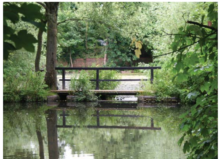
Figure 3.10 View across first pond to replacement bridge.
