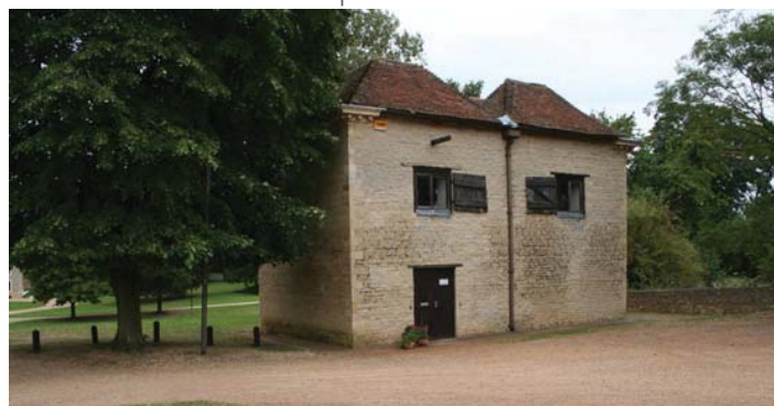
Figure 2.26 – showing the rear, unfinished elevation of the Pavilions
