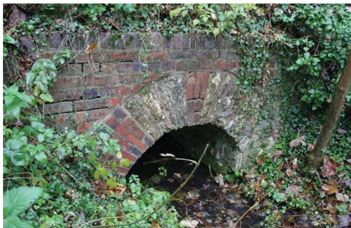
Figure 2.30 – the conduit, which formed part of the cascading water feature probably by Richard Woods
