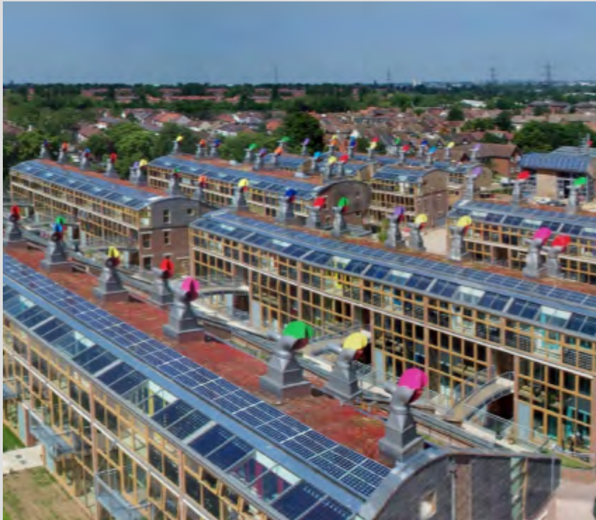
BEDZED zero-energy community (UK)
