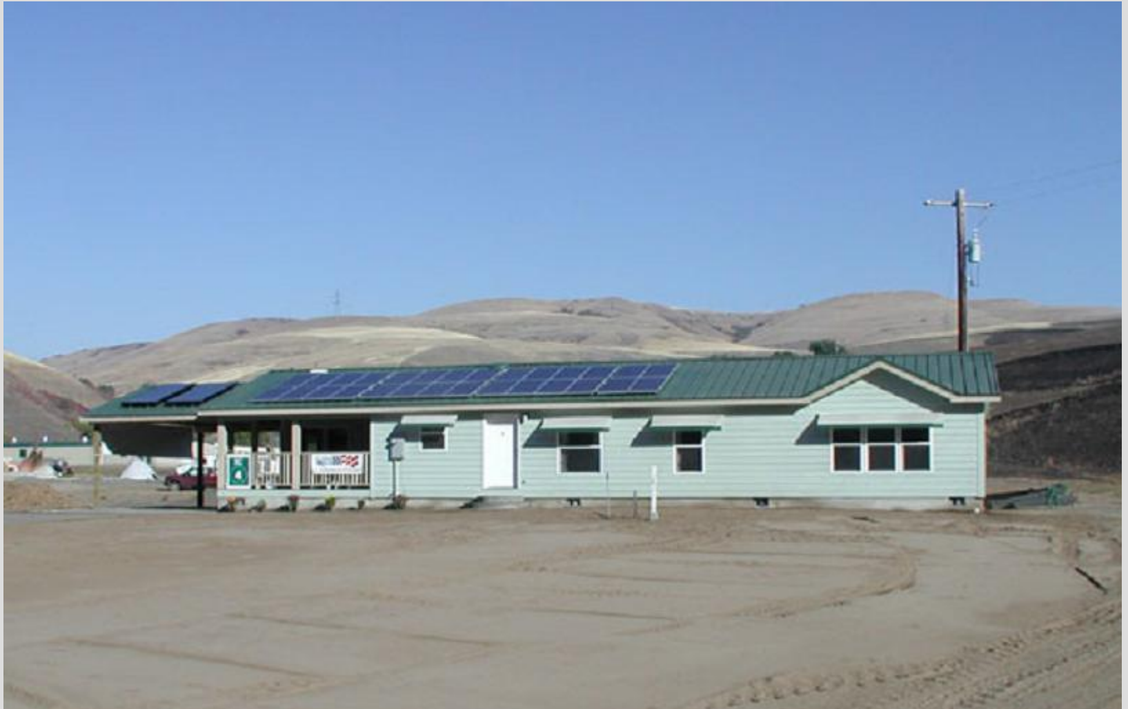
Nez Perce Zero Energy Manufactured Home Project
