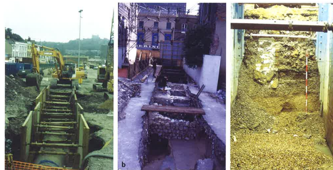
Figure 2.7a: View of sewer trench under excavation. Figure 2.7b: Excavated site. Figure 2.7c: End of trench for recording protected by trench boxes. All photographs by the author
