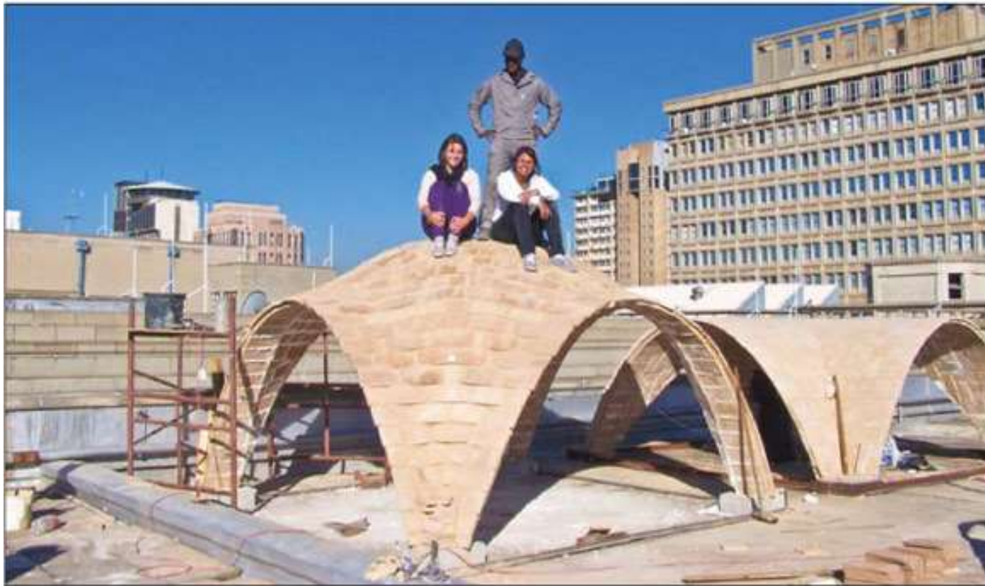
Figure 13 Completed shell and a demonstration of the structural strength
