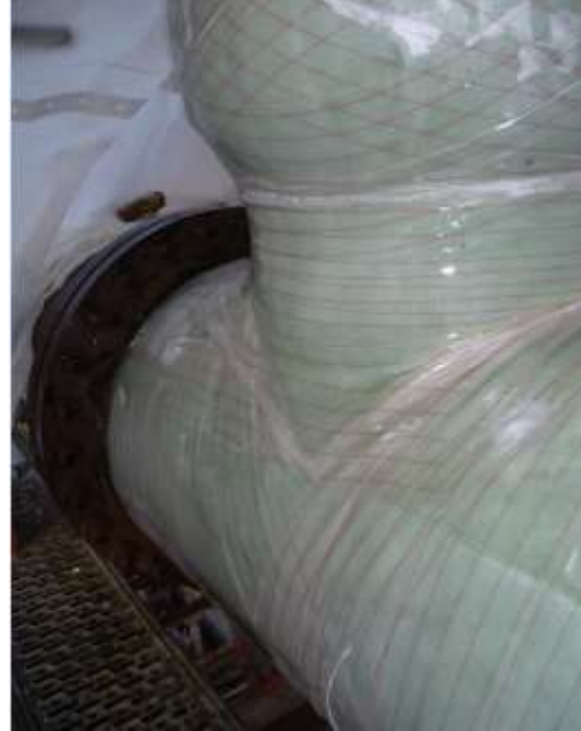
Figure 15: Composite Wrap Installed
