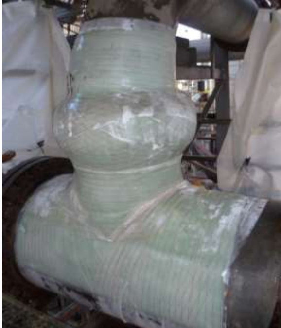
Figure 14: Composite Wrap Installed
